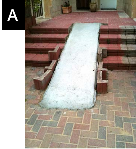
[Image description: A concrete ramp lays on top of a flight of stone outdoor stairs]
